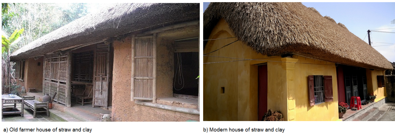
Figure 4. House of straw and clay - past (source photo left: Bao Moi (2017) and present (source photo right: Manh, 2016)
