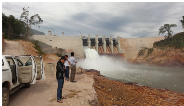
Figure 1. Survey in hydropower plant Theun Hinboun
